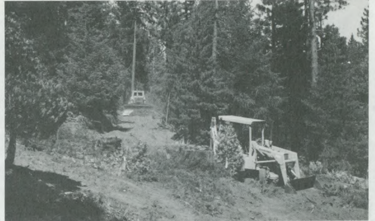
Workers prepare the sanitation-system drain field at Leoni Meadows.
