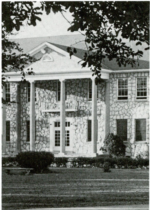
Oakwood College's J. L. Moran Hall now is used for classes but is familiar to alumni as the former administration building.
