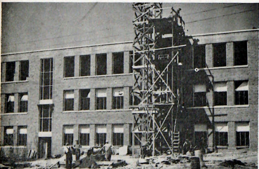
Look how it has grown! (Rear view of new science building)
