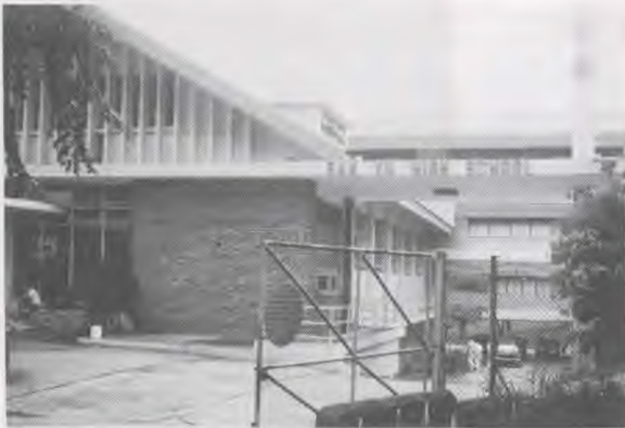
San Yu High School with the completed four-storey wing in the background.
