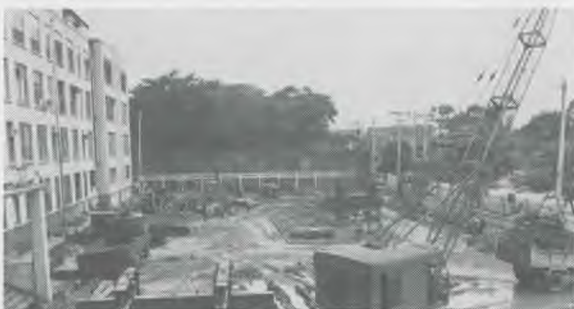
Construction of bore pile being done.
