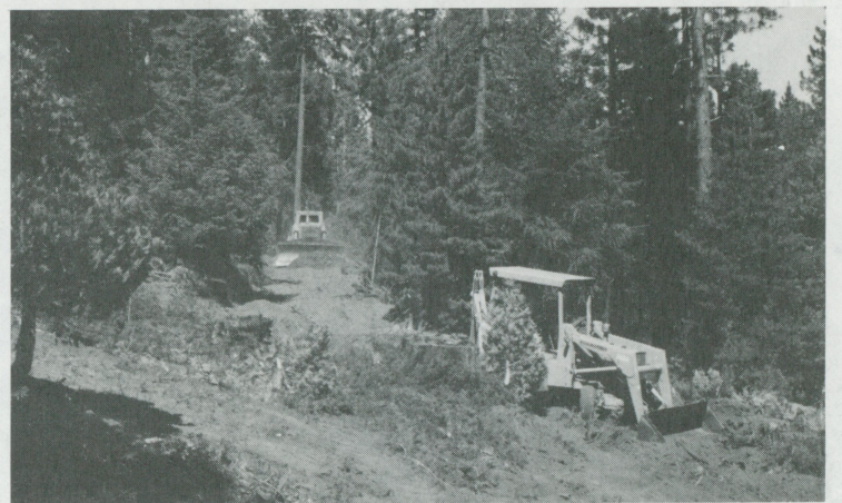
Workers prepare the sanitation-system drain field at Leoni Meadows.
