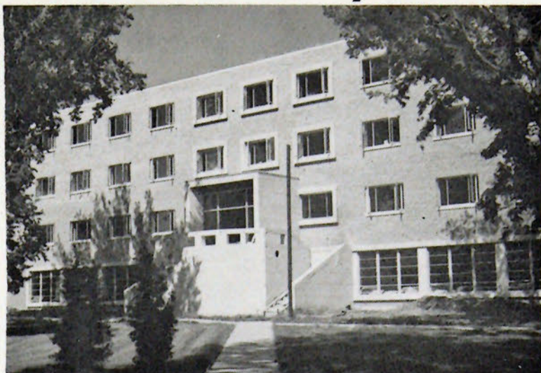
Here is South hall today. A steel and concrete, 3-story structure which at present has 95 student rooms and two lounges. The dining room is on the lower floor. The building is now L-shaped, but another wing is to be added making it U-shaped. The kitchen will be between the two wings.
