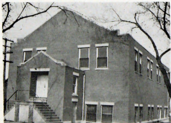
The gymnasium was a faculty-student project. With two faculty members in charge of construction, the students did the work and raised the money for materials. A swimming pool was dug under the building and the same pool is now in use though the structure has been changed.
