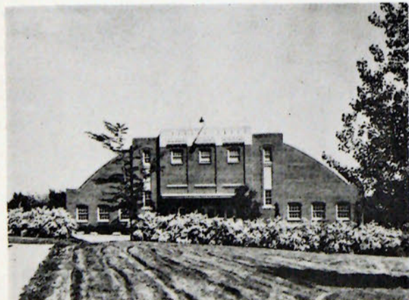
Expansion of the physical education department and increase in enrollment made the need for a large auditorium great. The 88 x 174 ft. building pictured above is used for Sabbath School, various programs, skating and regular gymnasium activities. A new scoreboard is the latest addition to this building.
