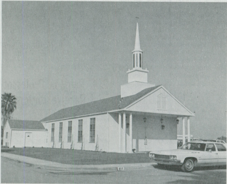
Exterior of the Blythe church is typically Colonial.
