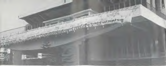
Kai Chek Chon Hall, site of the Word of Life Crusade, is located on one of Bangkok's busiest streets.
