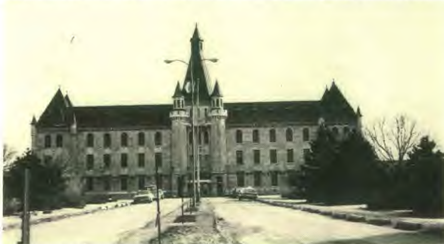
Collin's Bay Penitentiary, where a Five-day Plan to Stop Smoking was held March 17-21.
