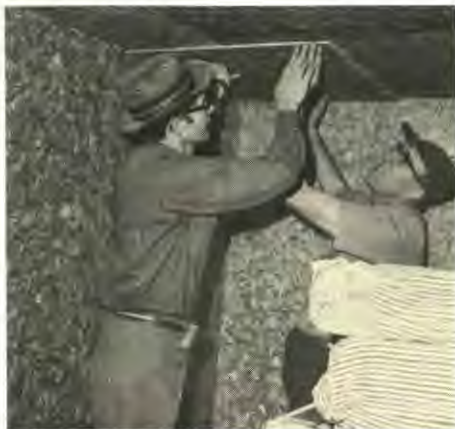
Ron Simanton and Pastor Littman sheeting in ceilings.
