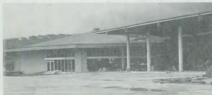
Construction continues on the Honolulu Central Church complex.
