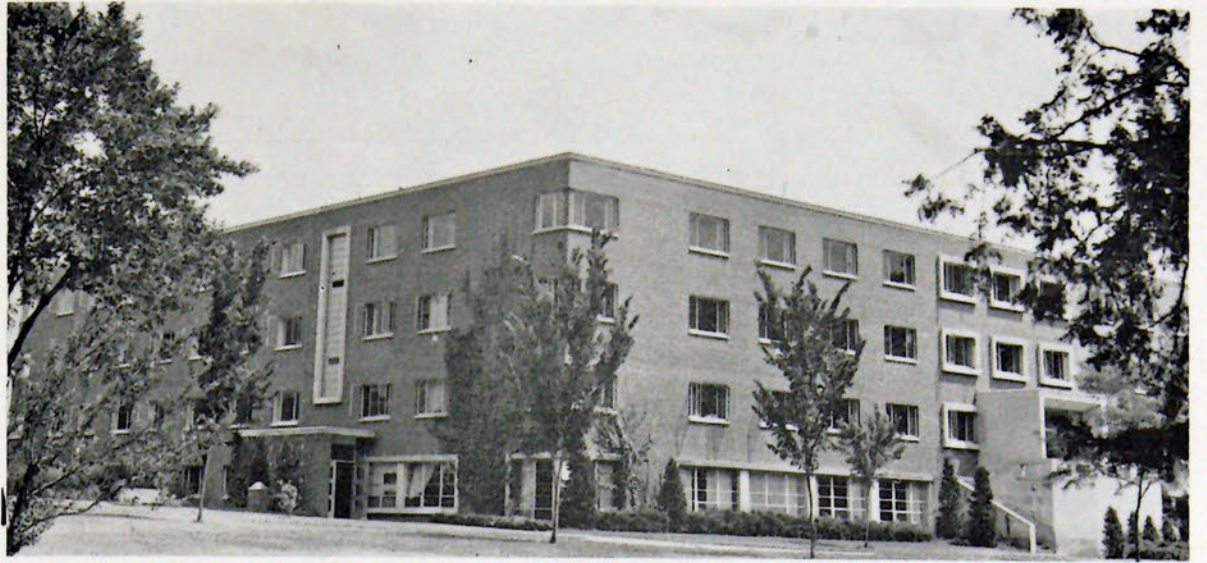
View of the new wing of South Hall, men's dormitory, which provides 46 new student rooms. This is part of the continuous building program designed to keep pace with Union's ever-increasing enrollment.
