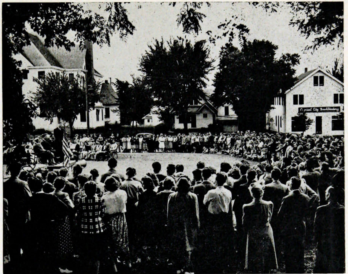
Ground-breaking exercises hold attention of students, faculty, and friends of the college gathered at the site of the new science building.
