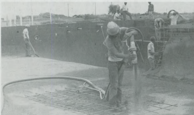
A workman nears completion of the base layer of concrete on the new swimming pool at TAA.
