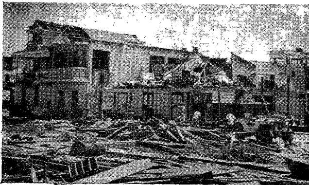
Hurricane destruction in Chetumal, Quintana Roo, Mexico, where only two buildings remained semi-intact.
