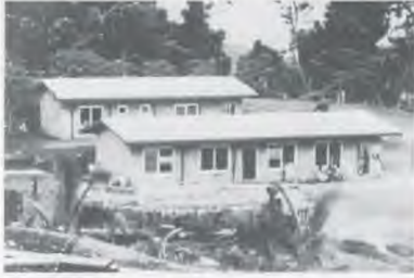
The building in the foreground is typical of the medical clinics to be built in the Solomon Islands with part of this quarter's Special Projects Offering.
