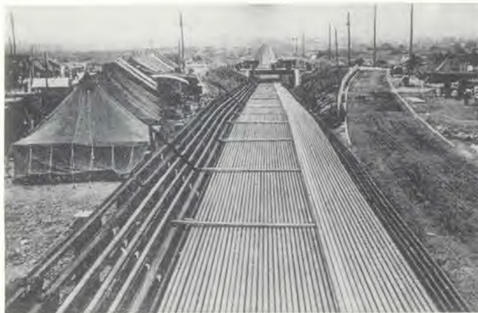
Two hundred miles of pipes which were laid under the English Channel to convey oil to the Continent during the Allied attack.
