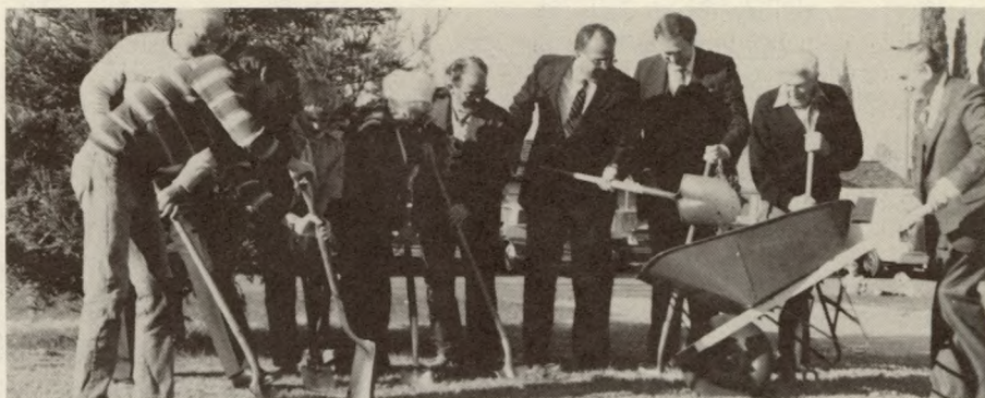
Richard Simons, the president of the Northern California Conference (fourth from right), breaks the ground at the Concord church's groundbreaking services and dumps the earth into Bob Burgess's wheelbarrow. Burgess, a member of the Concord church, is the building committee chairman for the new addition. Pastor Ed Allen is on the left.
