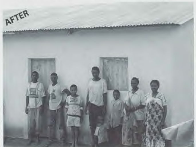
Covering the walls with cement plaster coating protects them from inclement weather; the coating process required more funds from ADRA Canada
