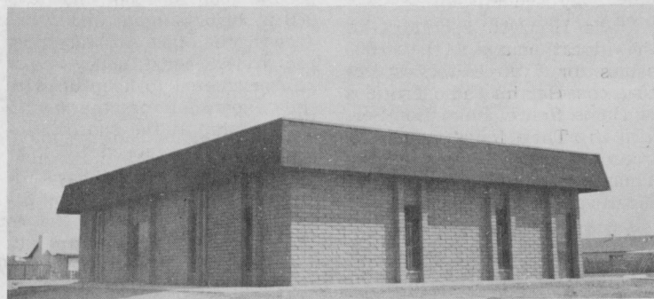
Maryvale members are now meeting in the completed educational wing of the proposed church complex.
