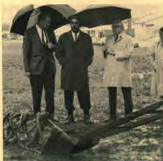
Alderman Frank Wansbrough, Milton Myers, building committee chairman and architect John Hreno decide that rain or shine the new Windsor Church will be built. The plough in the foreground was used to turn the sod.
