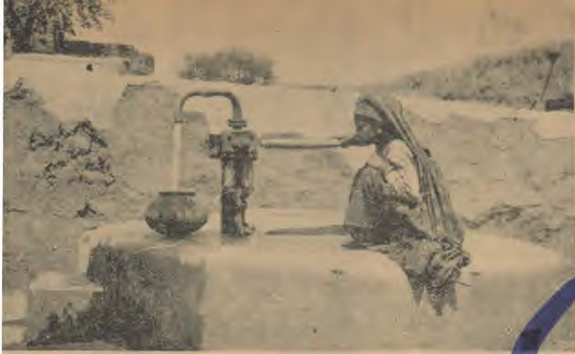
An improved village well, closed and provided with a pump.
