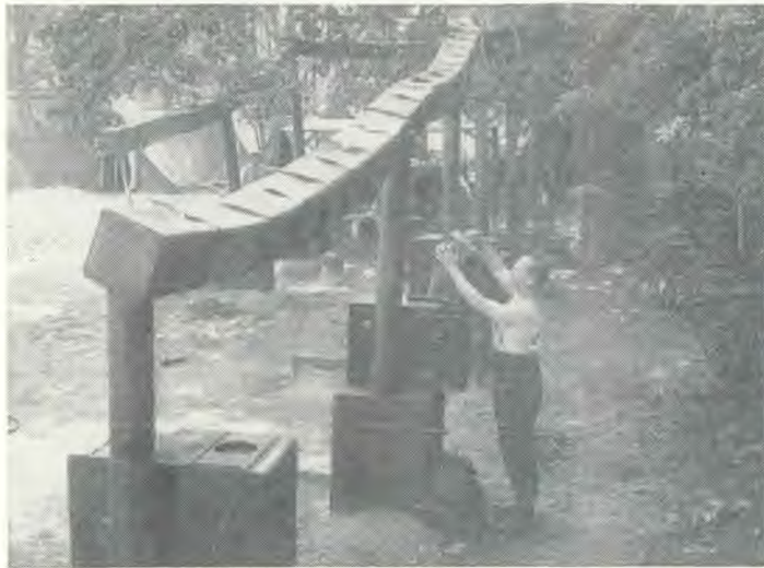
The R. A. F. cooks build an ingenious chimney of gasoline cans, which carries the smoke from the field kitchen into the nearby trees.
