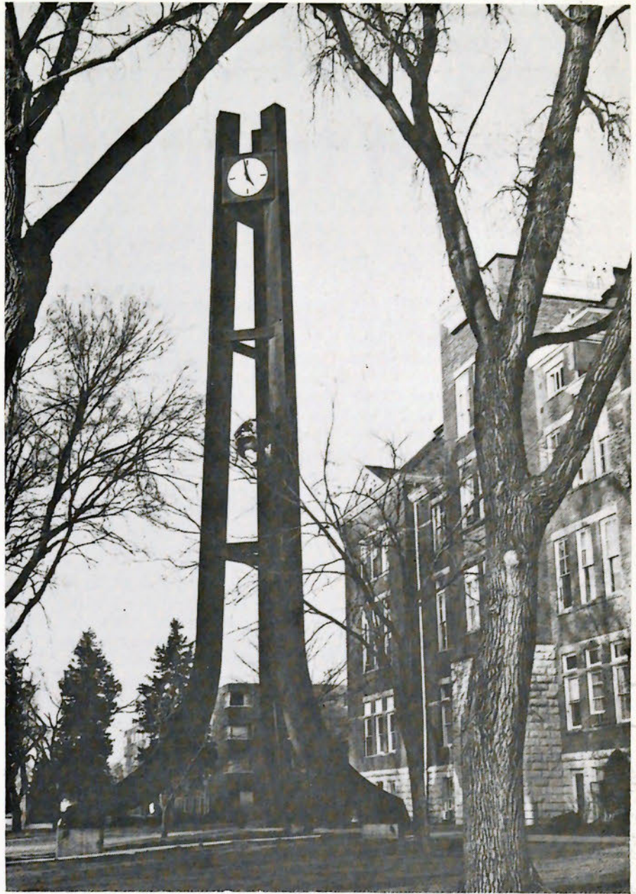
the new tower . . .
