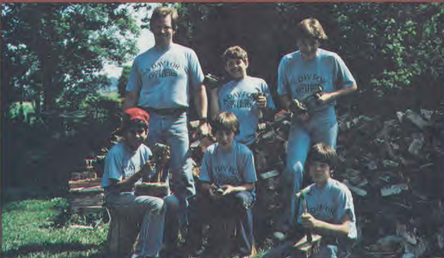
Brick-cleaning crew work on cleaning used bricks.
